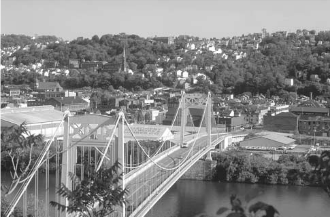
The Tenth Street Bridge and South Side Slopes
